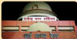
RAJENDRA NAGAR RAILWAY STATION 4.5 Km
